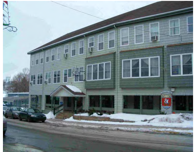
Figure 7.2 New Windows at Town Office
