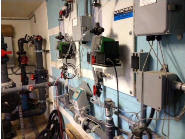
Figure 8.1 Upgrades to Wellheads (Process related -2013)
