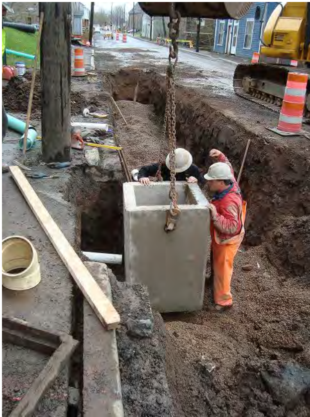
Figure 7.1 Installation of Main Storm Sewer Church Street
