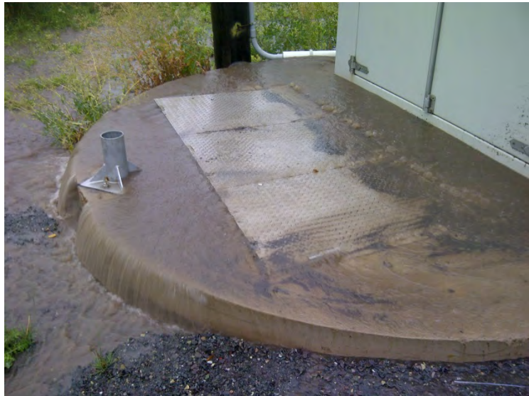
Figure 3.1: Pumping Station at Front Street
