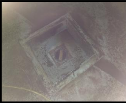
Drain on Floor of Water Tower Interior Before Refurbishment
