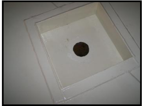
Drain on Floor of Water Tower Interior After Refurbishment
